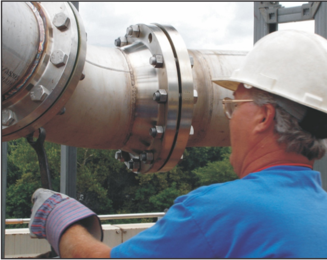
Installation of PSP® coated Schedule 10 pipe.
