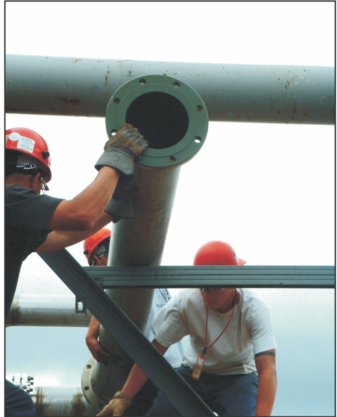
Aligning straight section of PSP® pipe.
