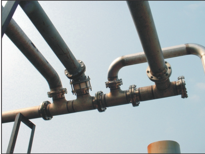
Completed installation of PSP® coated Schedule 10 pipe.
