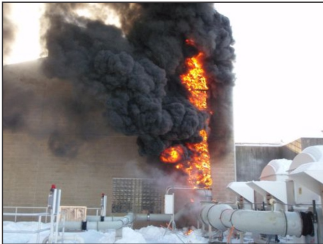
Estimated $1 million USD cost of fire damage to this wastewater treatment plant (FRP duct system).
