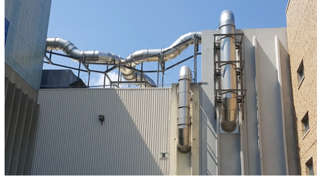
BioSolids and Dewatering Building.
