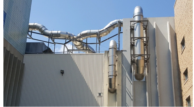
BioSolids and Dewatering Building.
