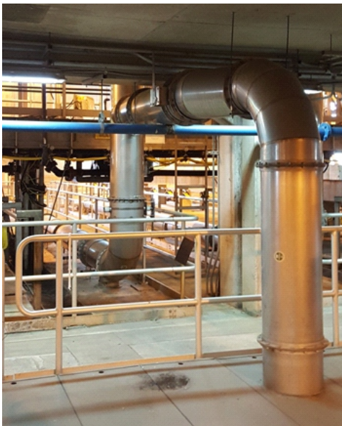
Coming up and across for Grit Chambers.
