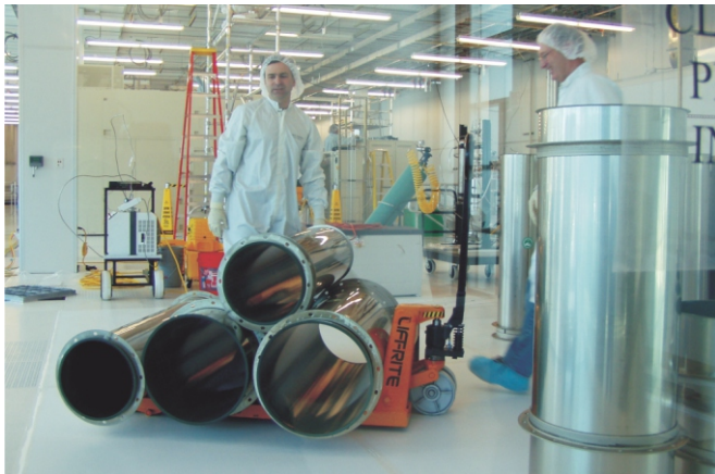
PSP® duct staged for installation by MCD Mechanical Contracting Technicians. Note clean room protocol is already in effect at this point of assembly.
