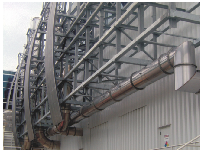
PSP® duct installed on exterior of NanoFab 300 North.
